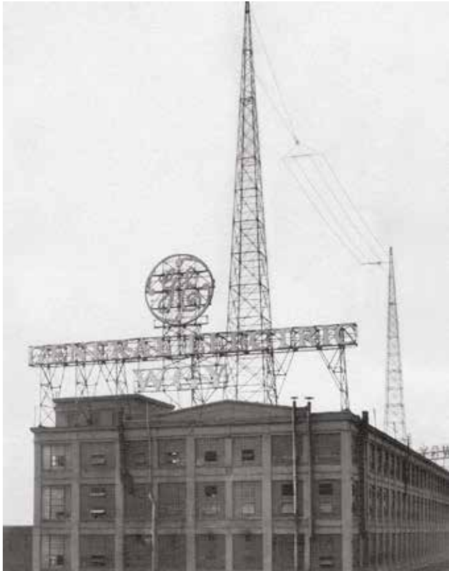
WGY's first antenna is seen on the roof of General Electric Building No. 40 in Schenectady. The two 183-foot support towers were spaced 350 feet apart, and the flat-top horizontal antenna was 200 feet long.
