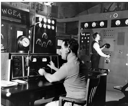
January, 1941 -- The 100 kW WGEO transmitter is at right; the older 50 kW transmitter at left broadcast for WGEA.
