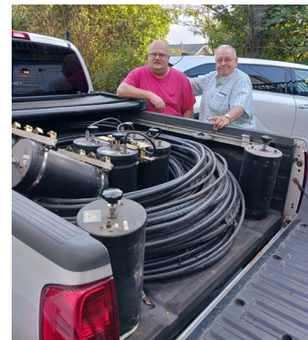
Walt and Steve take a breather after loading the coax and duplexers
