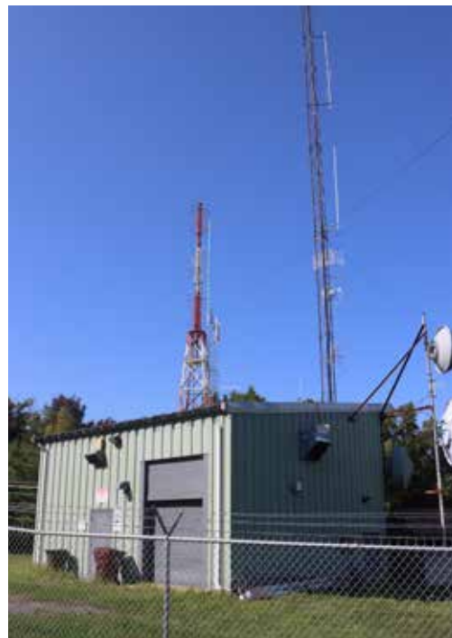
The 220 repeater is proposed for installation at the old analog site used by Channel 6, WRGB. The building currently houses the station’s digital backup transmitter and the transmitter of FM broadcast station WRVE.
