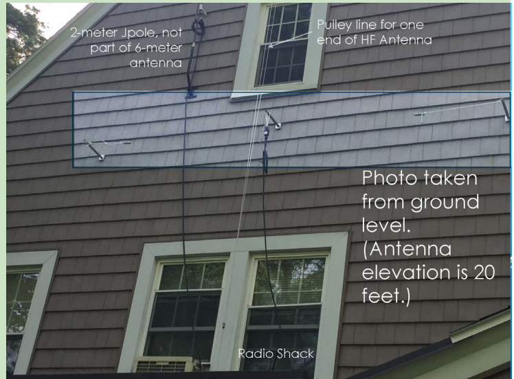
-- The finished project -- The highlighted area shows the three stand-offs for the 6-meter antenna.
