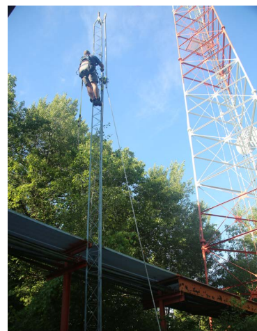
Bob Isby working on the current repeater antenna tower this past July.
