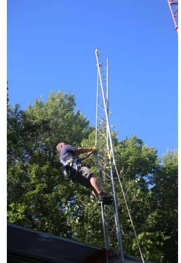
Bob skillfully raised each tower section into place using a "gin" pole.
