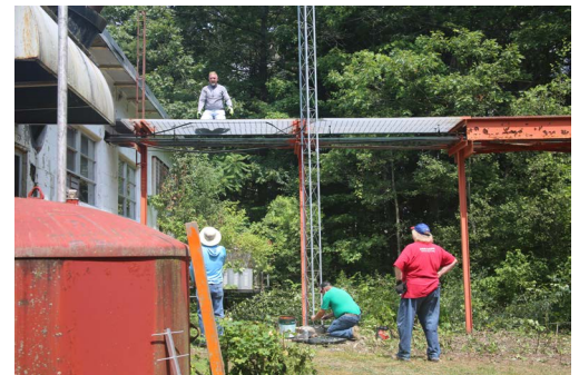
EGARA members finished up the install by grounding the tower, securing the coax line and running it to the repeater location inside the building.
