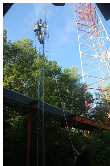
Bob Isby, K2RHI, hoists a tower section in place for the club's VHF repeater antenna. The old WTEN analog tower is in the background.
