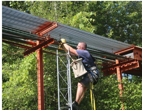
Tower Guru Bob Isby, K2RHI, secured the Rohn 25G tower to the old WTEN-TV coax bridge.
