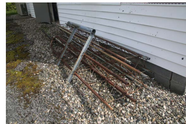
In early June, the club located used Rohn 25G tower sections for the project.
