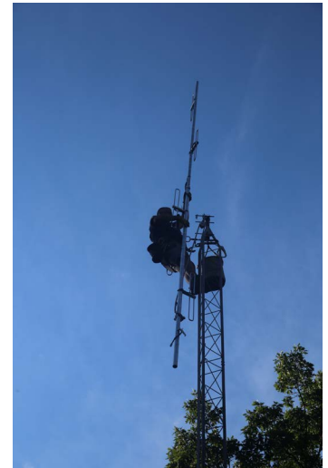
Bob finalizes the repeater tower project by preparing to mount the 4-Bay antenna to the top of the mast. Time from start to finish was about four hours.
