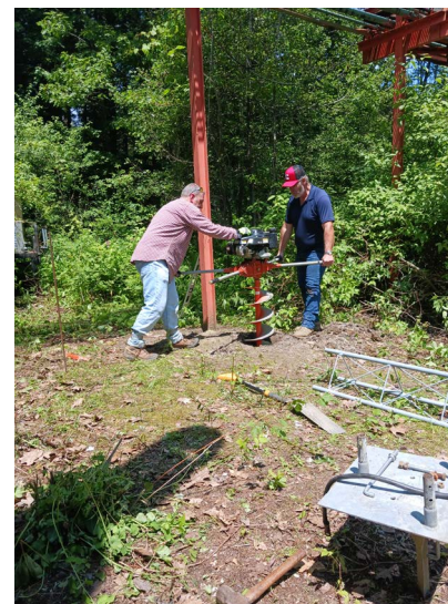
The long-awaited tower installation began with digging the footing for its base. Matt Saplin, W2SAP, and Pat Negus, W2PMN, handled the auger.
