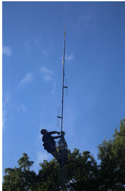
Bob bolted the 4-bay antenna in place and connected the coax feed line. The entire tower install was completed in just over four hours.
