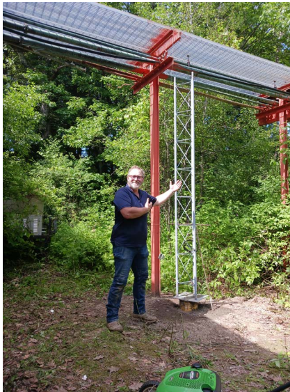
With the concrete set and the tower base in place, Pat Negus unveiled the first section to go up.
