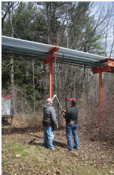
Work begins with Walt Snyder, N2WJR, and Pat Negus, W2PMN, making a survey of the proposed tower site and necessary measurements.
