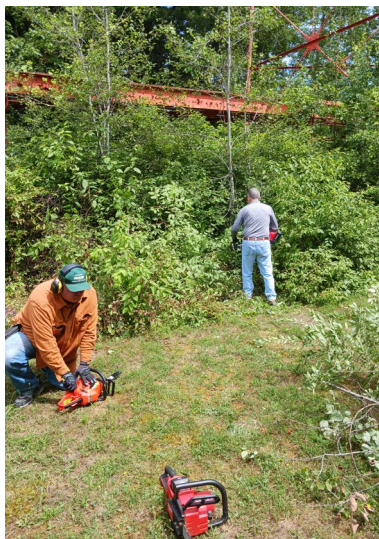
To prep the project, the old WTEN site was cleared of brush, trees and weeds, including the area under the coax bridge where the EGARA tower is secured.
